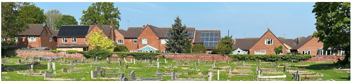
Brick wall with areas of thick ivy
